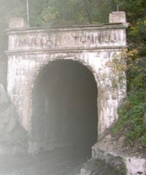
Completing the work in one season was now impossible, so preparations were made to get the tunnel through the winter. In some areas water continuously comes through the lining and runs in the drains. If the lining is not properly prepared and insulated, ice becomes a problem.
