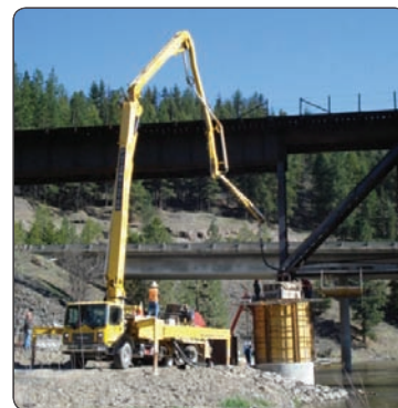
Above: Encasing the pier in concrete.
