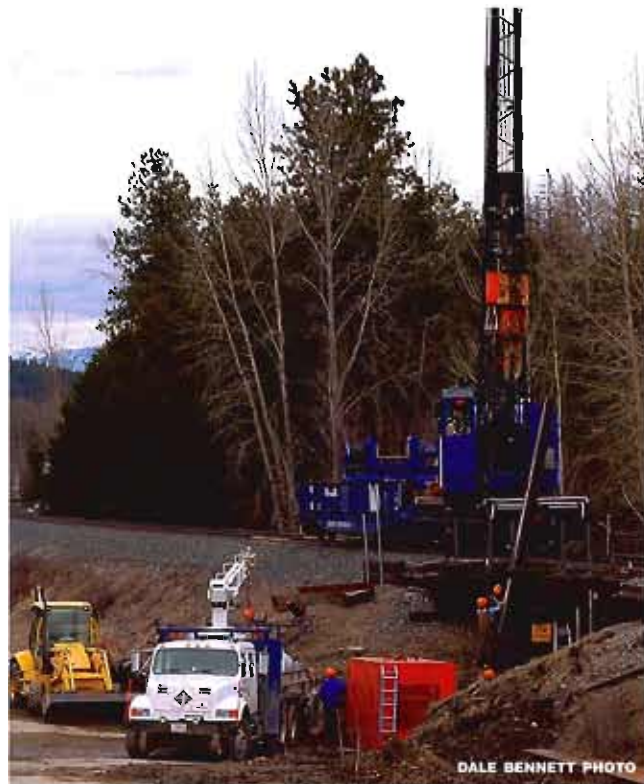
Bridge Crew 101807 is at work renewing Bridge 112 near Kootenai, Idaho. Pictured here MRL locomotive crane 100411 and pile driver, operated by Tom White , vibrates steel pilings. The new 60-foot, four bent ballast-deck bridge replaces a timber structure. Completion is slated for mid-May.
