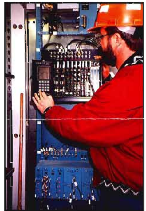
▲ Dale Smith, assistant signal and communication supervisor, checks the crossing processor equipment at a crossing signal installation near Missoula. Milt Clark photo.
