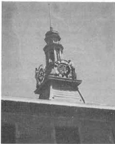
Doug Thomson and Rich Labbe install new hands on the depot clock (a Seth Thomas, ca. 1903) at Helena.
