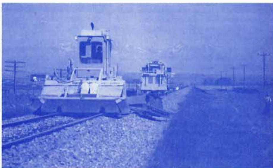
Guided by beams of light, the Jackson 6700 tamper (in distance) aligns and smooths the main line east of Big Timber on May 25, 1988. A ballast regulator follows going back and forth to redistribute ballast uniformly along the track and into the crib areas between the ties.
