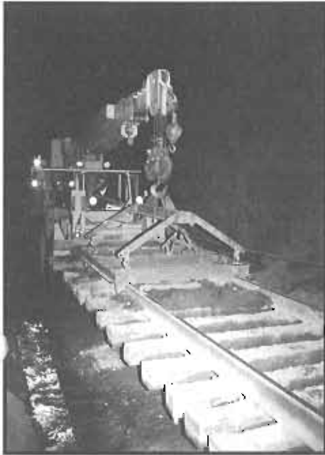
Old track panel being removed.
