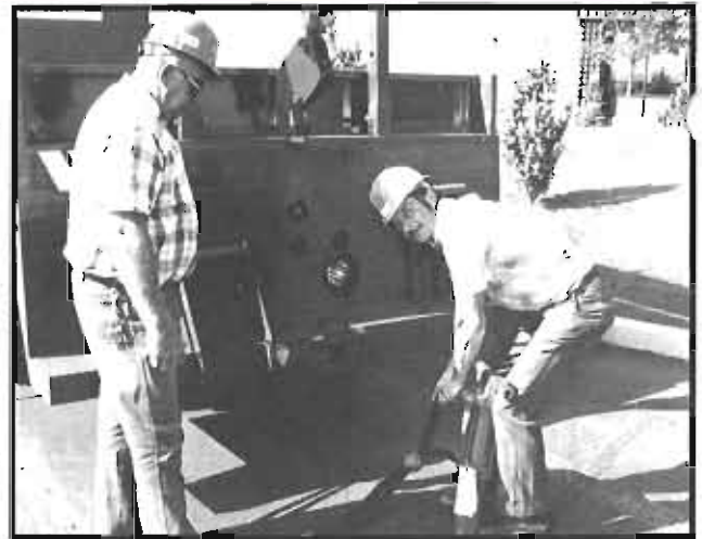
The Super Truck for the Plains, Montana, Section Crew fresh from the Equipco shop on September 6 where the tag axle, other accessories, and the markings were added. Right, assistant roadmaster Don Boltz and Plains truck driver Gary Baltz demonstrate the operation of a hydraulic spike hammer.
