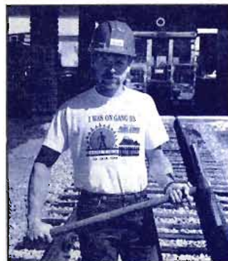
Gang 53 installed a MRL record-setting 2,100 cross ties during one 10-hour shift on May 23 near Perma, Montana. Commemorative T-shirts were given to the gang members. Pictured here, machine operator John Harbrige is wearing one of the, sure to be, collector's items.
