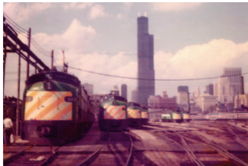
Looking northward into 'B' yard from the main crosswalk. It's a latespring afternoon in 1976. Serviced locomotives and trains wait for their crews to back them into Chicago Union Station for the evening parade. Photo by Dennis Popish.
