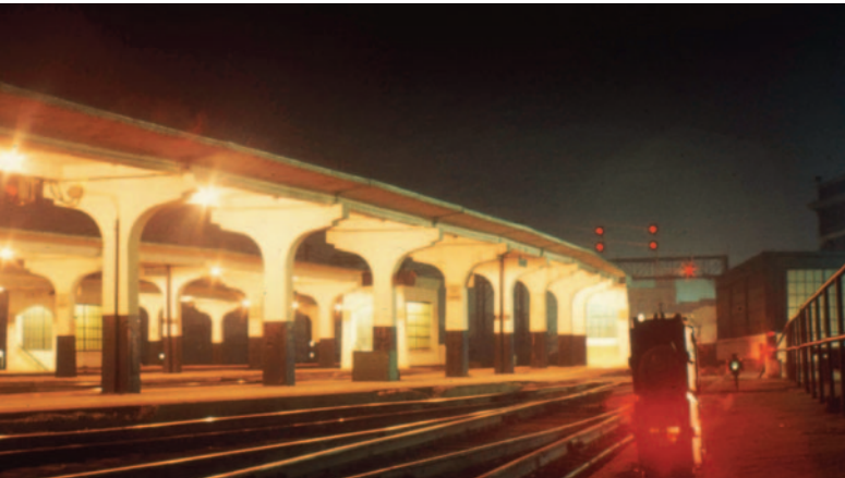
The Aurora coach yard and passenger platforms are empty early in the evening of Nov. 30, 1973, but will soon start to fill as west-bound dinkies start arriving. The station is on the right. Photographer unknown, from the Leo Phillip collection.
