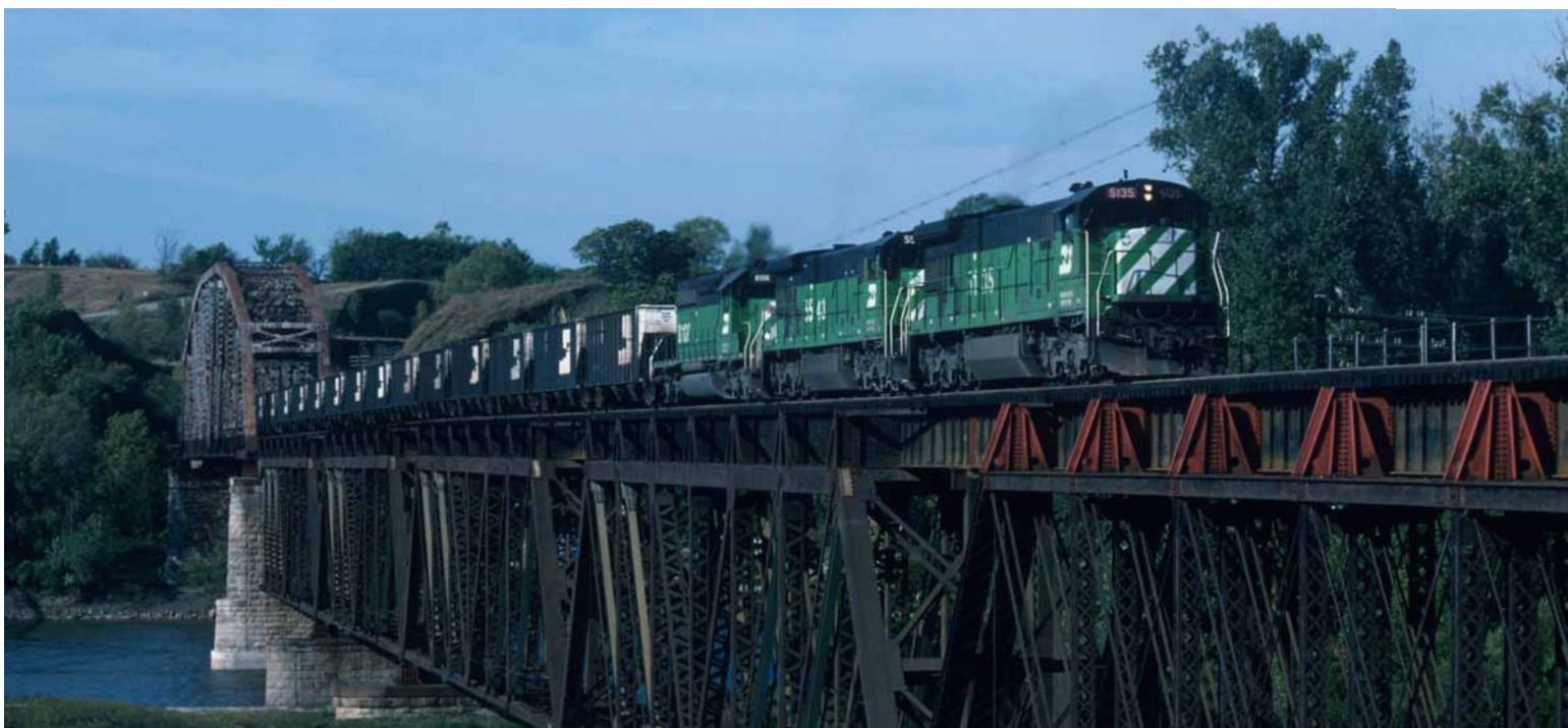
An eastbound loaded coal train crosses the approach portion to the main span of the first bridge on September 30, 1993. Photo by David P. Oroszi.
