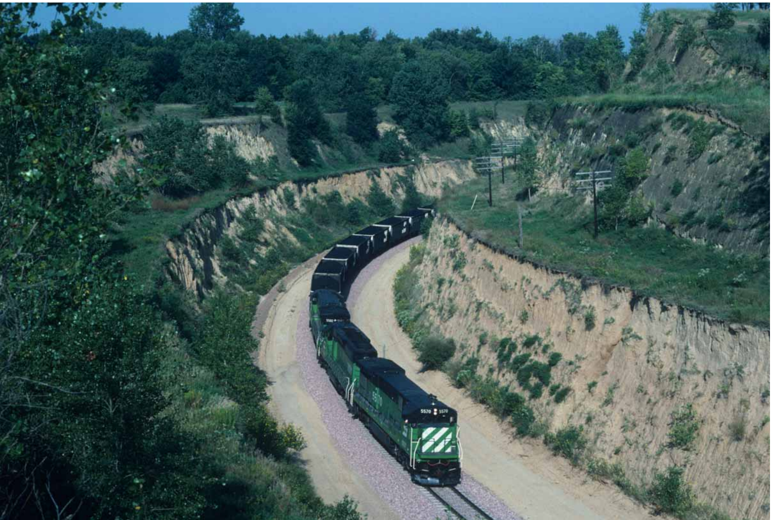
A loaded eastbound coal train glides through the cut just west of the bridge. Considerable erosion, a harbinger of things to come when the lower step of the cut was removed to make room for the second track, is visible on the left (south) side of the cut. September 1, 1990. Photo by David P. Oroszi.
