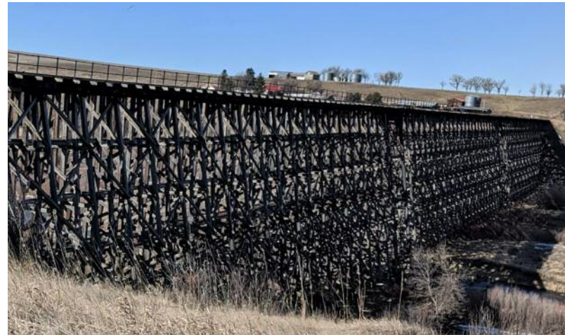
The out of service trestle over Big Spring Creek in March of 2020. Being built of wood, fire was an ever-present danger, especially back in the days of steam. To avoid complete destruction, the bridge is divided into three sections with an all-steel span separating them. While still devastating, only a third of the bridge would have to be repaired if a fire broke out. Photo by Bridget Demaline.
