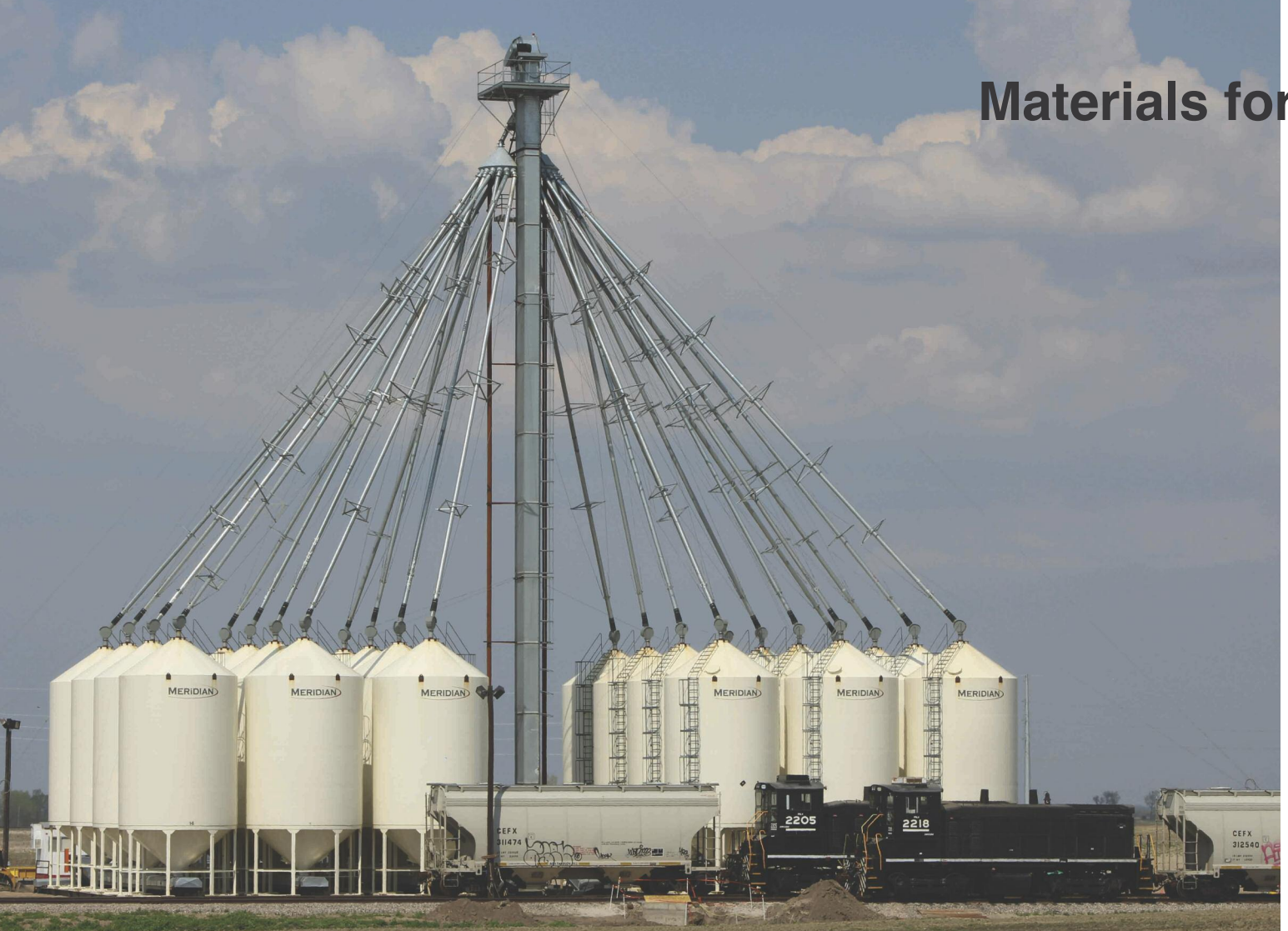
The frac sand facility at Berthold, just north of Hwy 2 on the Crosby branch. It can unload 100 cars a day and has storage capacity for 6,600 metric tons. It employs two EMD switchers which appear to be former NS SW1500's. May 26, 2015, photo by Micheal Farley.
