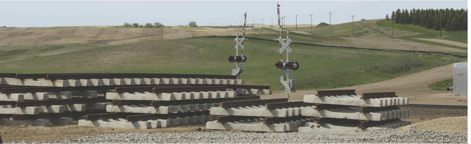
New panel track is awaiting installation at the crossing just west of Ross causeway at CP 635. May 26, 2015, photo by Micheal Farley.
