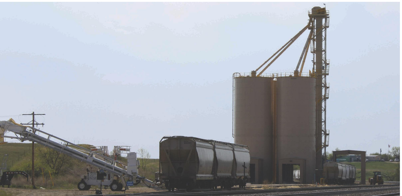
The frac sand facility at Blaisdell. Sand is loaded directly from hopper car to truck using the portable loader on the left. Sand is also unloaded from hopper cars and stored in the large silos for future loading into trucks. May 26, 2015, photo by Micheal Farley.
