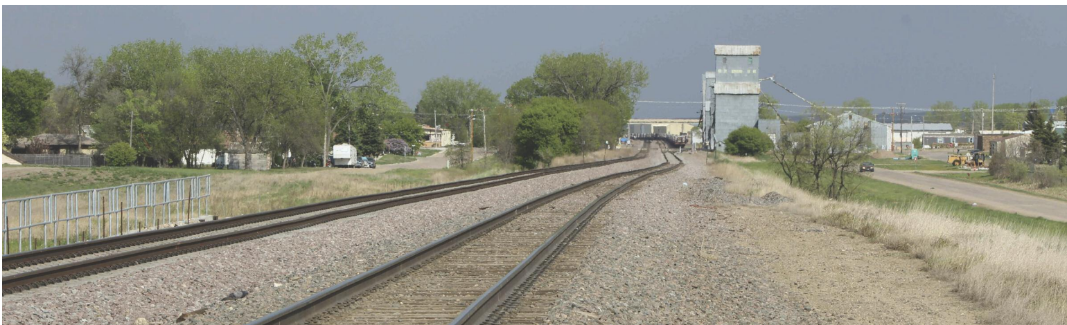
An example of a main line jog, here looking east towards Tioga. The existing mainline is on the right in the foreground, and left in the background. The existing main track was cut and realigned here resulting in the jog. This will also need to be done between Des Lacs and Lonetree, since the new Des Lacs River bridge is south of the existing structure, while the new track at Lonetree is north of the existing main. Another example of a jog will also exist just west of the Ross causeway. May 26, 2015, photo by Micheal Farley.
