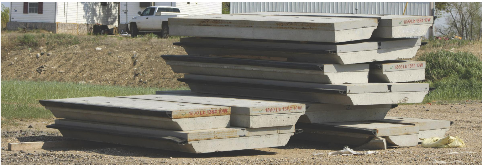
New tracks means new grade crossings. Parts for a new crossing (below) await installation at Blaisdell (above). May 26, 2015, photo by Micheal Farley.
