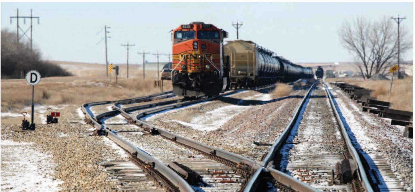
(below) Two long storage tracks each capable of holding 120-car unit trains branch to the left off the Zap Line main.
