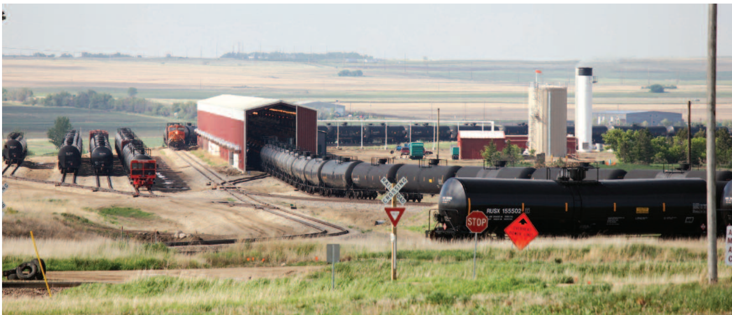
(above) The loadout, storage tracks and part of the loop are visible in this photo looking south from just off Highway 8. Note the bright red Nordco Shuttlewaggon mobile railcar mover on the first storage track left of the loadout.
