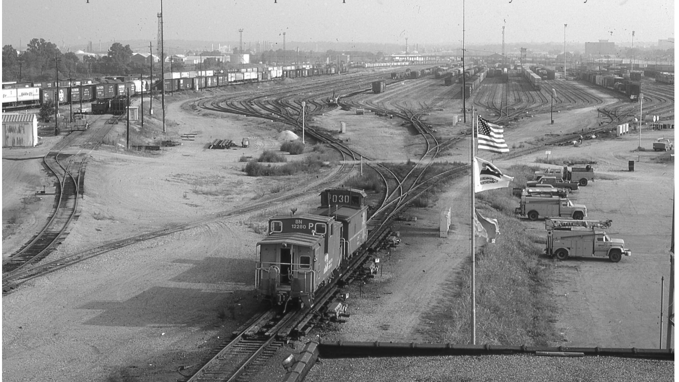
BN and Santa Fe cabooses slide through the retarder and into the bowl of the Cherokee hump yard on August 21, 1982 as seen from the platform outside the office at the top of the hump tower at the south end of the yard. Photo by Mike Condren.
