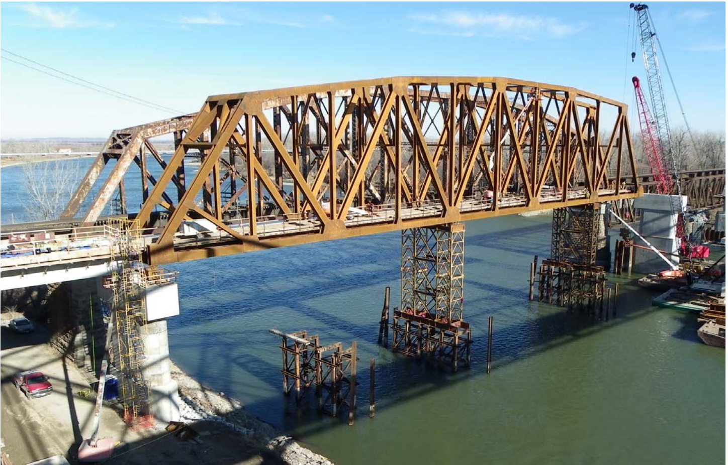
The through-truss portion, on the west (Nebraska side) is very close to reaching the middle river pier. Once that is completed, the base and deck work will begin on the east half of the bridge, using steel plate girders. View is looking northwest from the U.S. Highway 34 “Toll” bridge.
