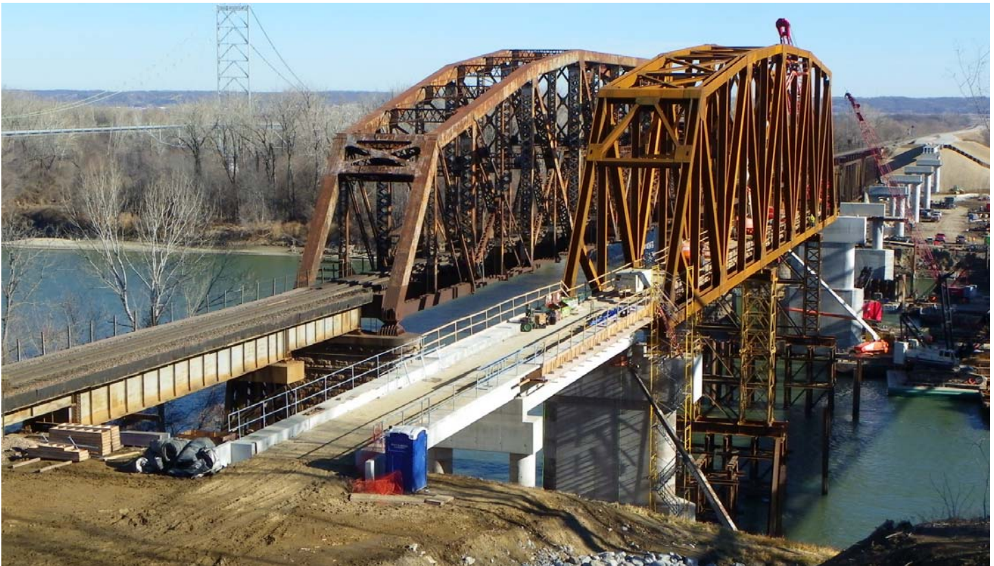
The through-truss portion, on the west (Nebraska side) is very close to reaching the middle river pier. Once that is completed, the base and deck work will begin on the east half of the bridge, using steel plate girders. View is looking northwest from the U.S. Highway 34 “Toll” bridge.
