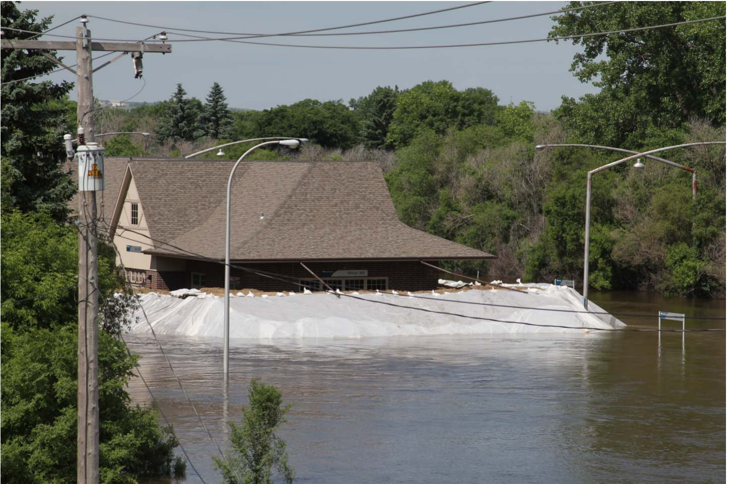
A berm was constructed around the Amtrak station in Minot to keep it dry. After the flood waters receded, it was a broken water pipe that kept it closed.
