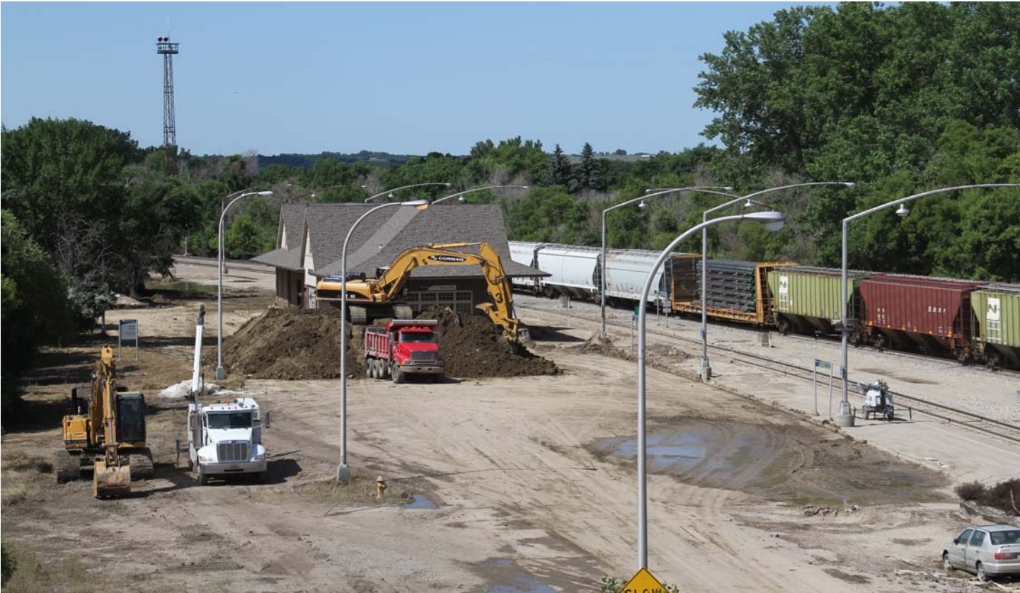
A berm was constructed around the Amtrak station in Minot to keep it dry. After the flood waters receded, it was a broken water pipe that kept it closed.
